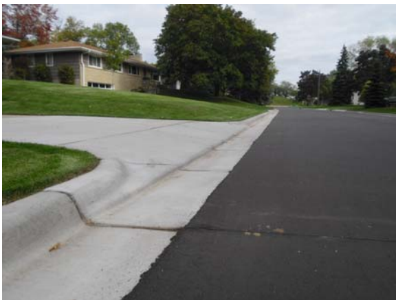
Barrier Curb and Gutter
