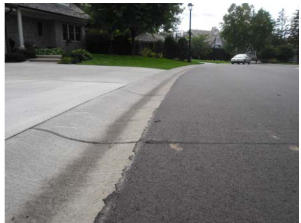
Surmountable Curb and Gutter
