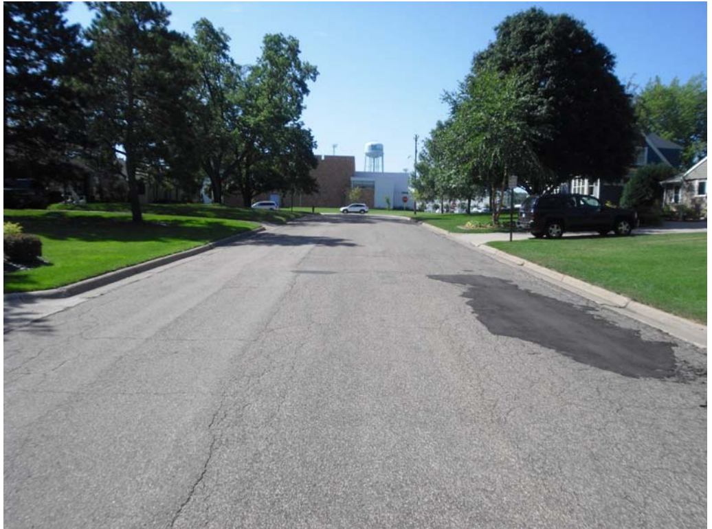
Photo 2. Existing Pavement Condition
