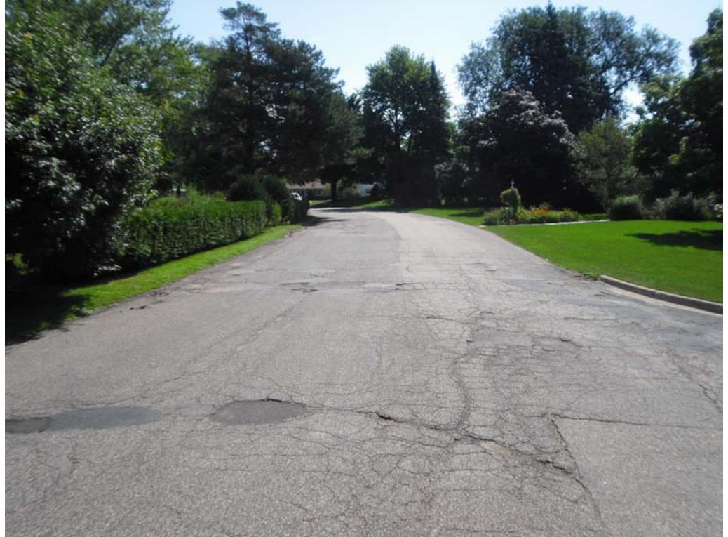
Photo 1. Existing Pavement Condition
